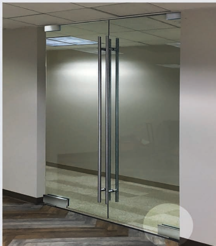
A-style Doors with Closer/fitting & Top Patch Fitting
