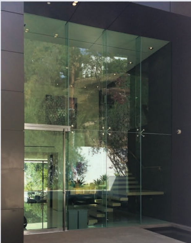
Glass Wall System with 3/4 Clear Tempered Glass
