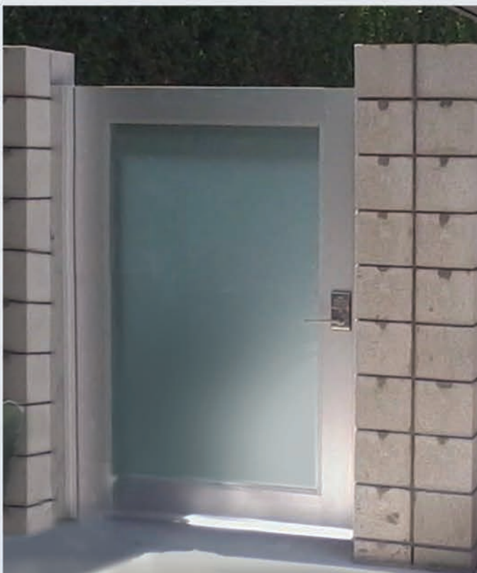
Aluminum Gate with Acid Etch Glass
