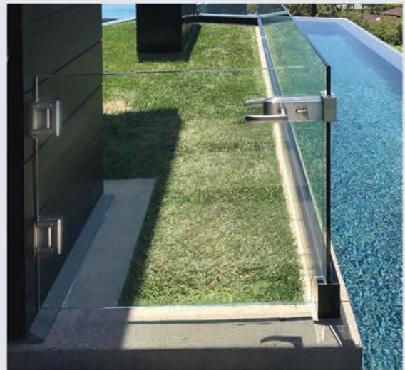
Security Gate with Custom Strike Application
