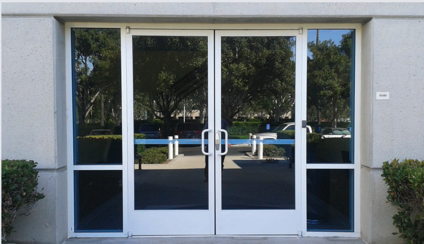
Double Aluminum Doors with Reflective Glass, Panic Hardware & PL-3 Offset Pulls
