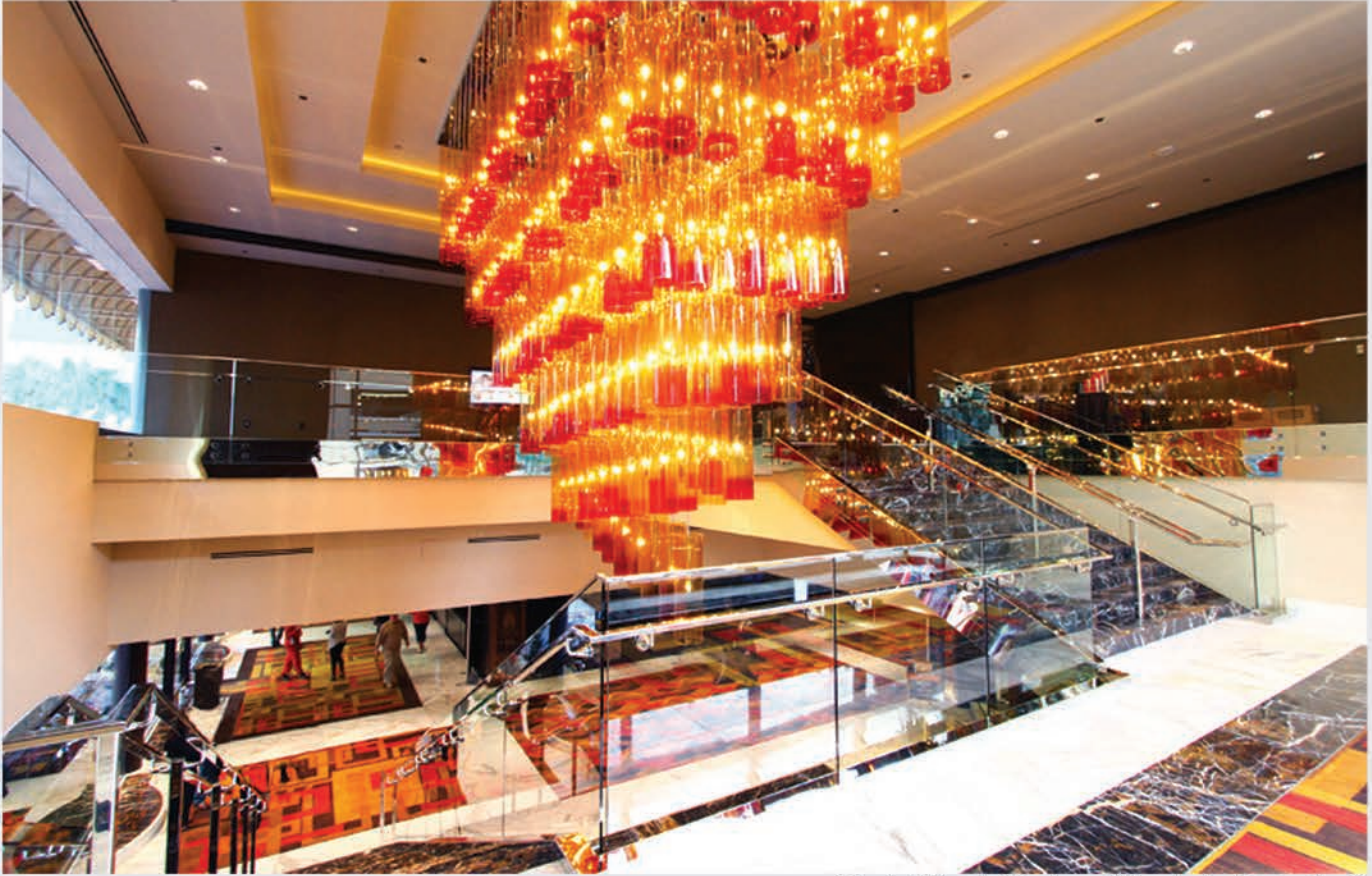
Stand-off Handrail System with Laminated SentryGlas®
