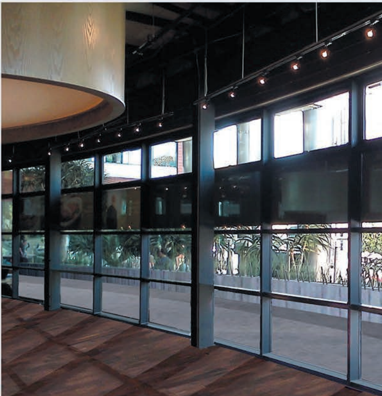
Curtainwall System with Reflective Glass
