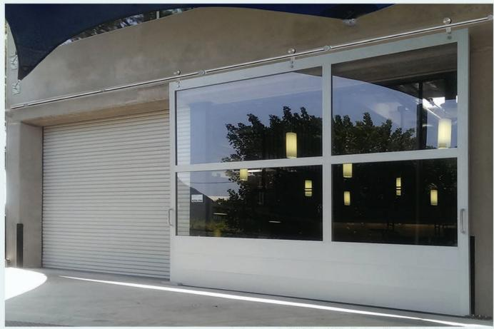
Custom Oversize Wall Mount Slider System with a Max Aluminum Slider Door
