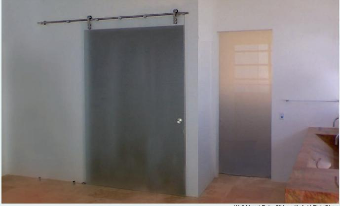
Wall Mount Ruby Slider with Acid Etch Glass
