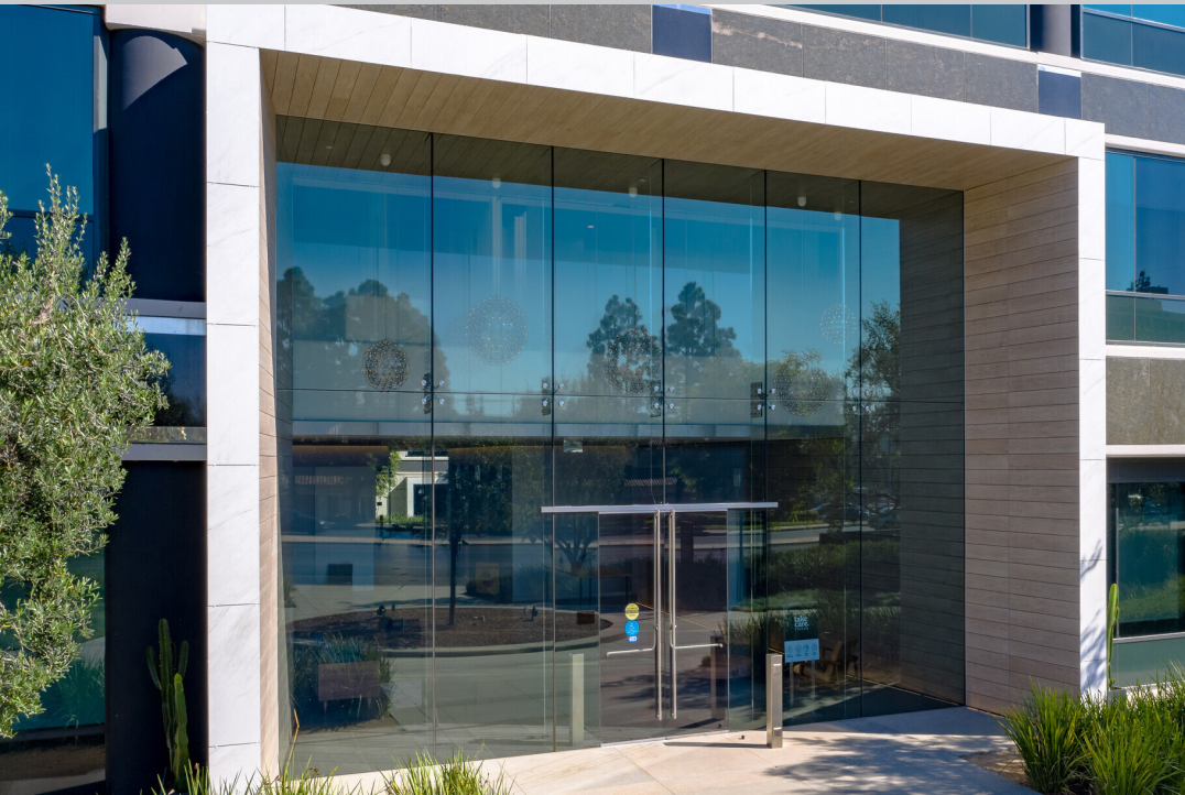
Frameless Tempered Glass Entrance Door System
