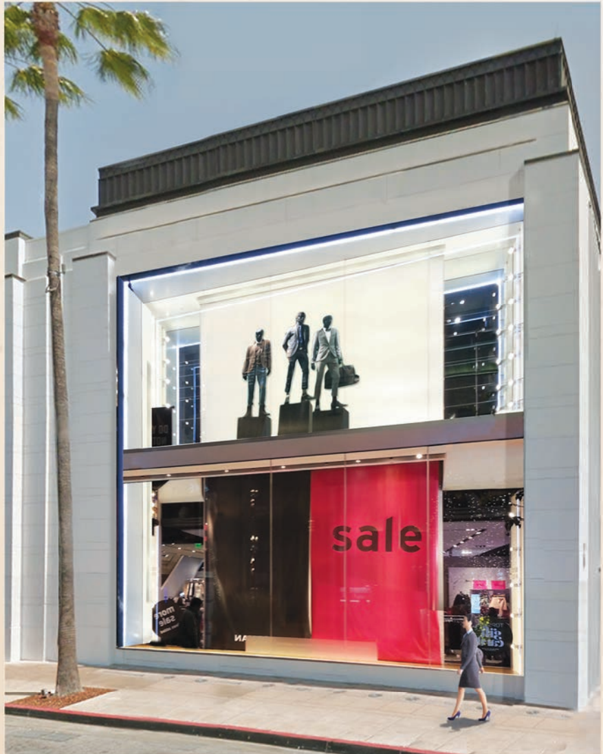
Oversize Fixed Panel with 3/4" Tempered Glass
