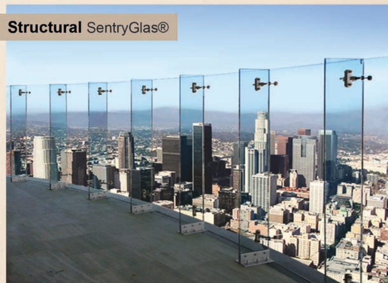
Structural Safe Laminated Glass with Custom Brackets & Spiders
